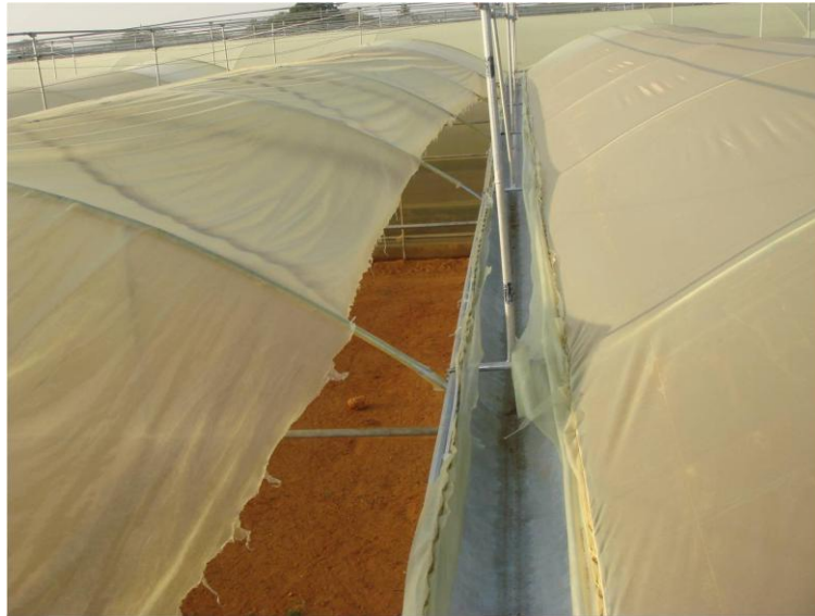
Damaged Plastic in a new greenhouse due to sharp profile
